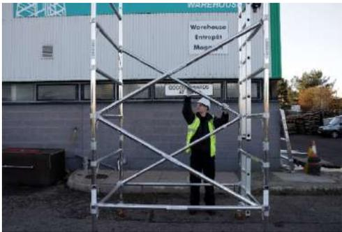
5. Add 4 diagonal braces from the 1<sup>st</sup> to 3<sup>rd</sup> and 3<sup>rd</sup> to 5<sup>th</sup> rungs as shown, level the tower using a spirit level as a guide.
