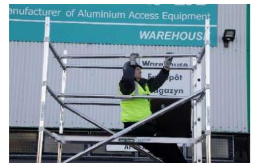
8. Climb the ladder inside the tower and sitting through the trapdoor fit 4 horizontal braces face down onto the 1<sup>st</sup> and 2<sup>nd</sup> rung above the platform to form your guardrails, as shown.
