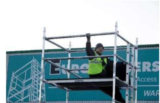
12. Climb the ladder inside the tower and sitting through the trapdoor fit 4 horizontal braces face down onto the 1<sup>st</sup> and 2<sup>nd</sup> rung above the platforms to form your guardrail braces as shown.
