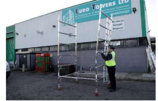
4. Fit the next set of frames onto the base, ladder frames run continuously up the left hand side. **Note:** see kitting page for frame
