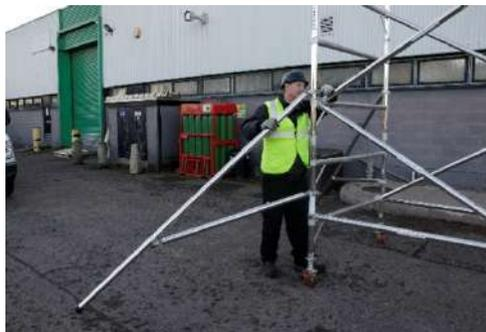
6. Fit the 4 stabilizers supplied with your tower. **Note:** Always fit 4 stabilizers unless building in a corner, inner stabilizers fit parallel to a wall. See kit list for correct size required to build your tower.
