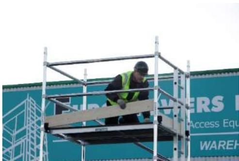
13. Fit the toeboard clips to the rung next to the corners of the platforms and then fit the toeboards as shown.
