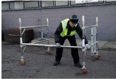
2. Fit one horizontal brace on the plain side of the frames to the vertical of the frames above the 1<sup>st</sup> rung connecting the 2 frames together.
