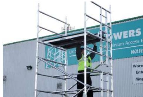
11. Fit the plain platform followed by the trapdoor platform 4 rungs above the one you are standing on. **Note:** There must always be 2 rungs clear above any platform so you can fit safe guardrail braces.
