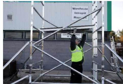
7. Fit a trapdoor platform to the 4<sup>th</sup> rung, trapdoor to the ladder end. **Note:** Platforms are positioned every 4 rungs.
